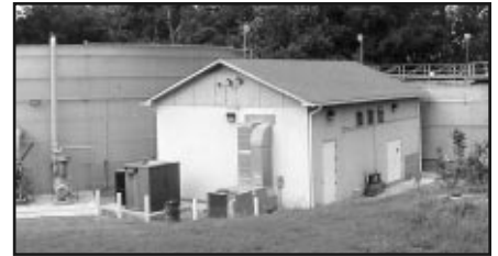
Figure 1. Side view of Reactor 1.
