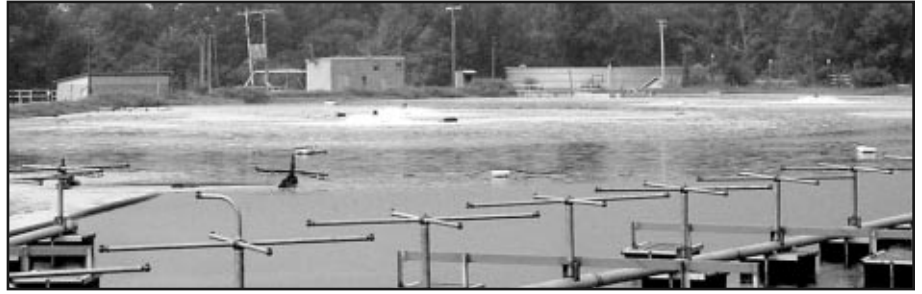
Figure 3. A portion of the fresh water pond with treatment plant in back right of photo.
